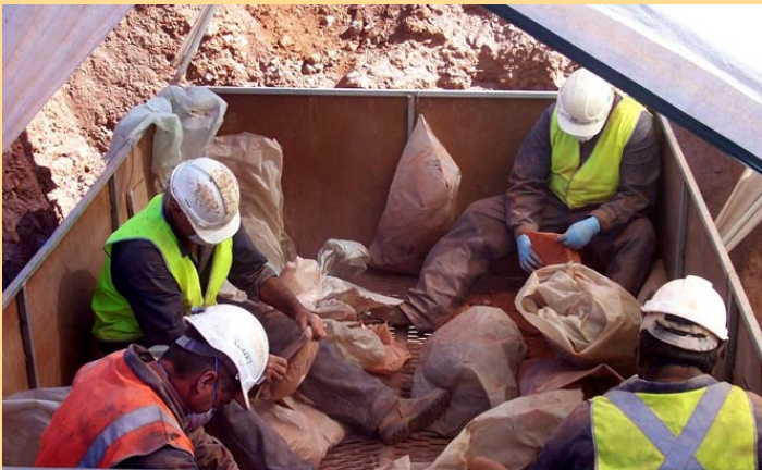
Above and below: Contractors and Marathon field staff systematically retrieve and empty bags of drill cuttings buried in an unauthorised pit at Mount Gee.
