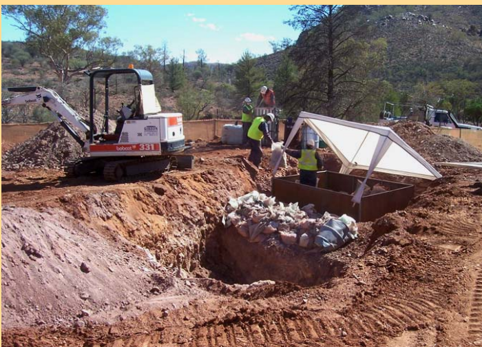
Above and below: Contractors and Marathon field staff systematically retrieve and empty bags of drill cuttings buried in an unauthorised pit at Mount Gee.
